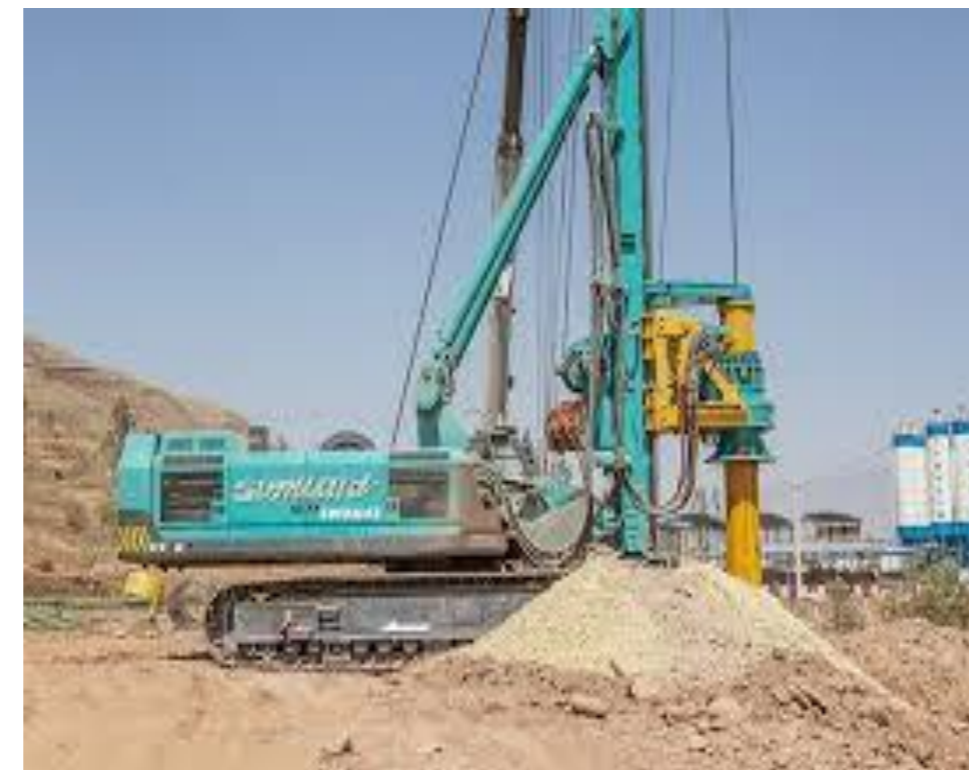
FOUNDATION DRILLING RIGS
