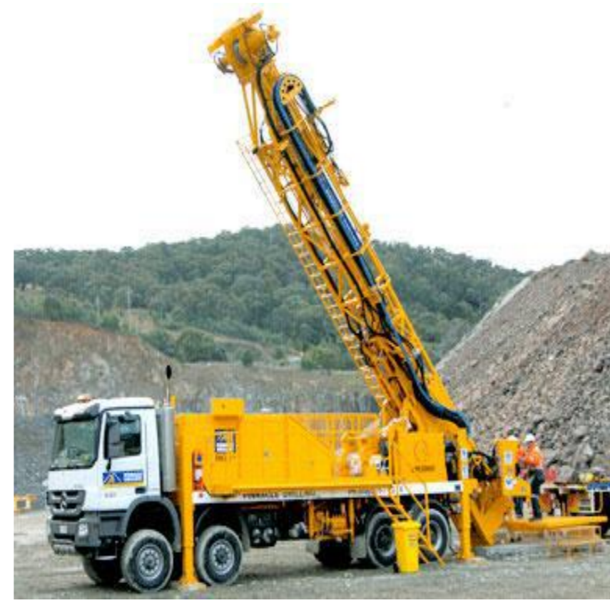
CORE DRILLING RIGS
