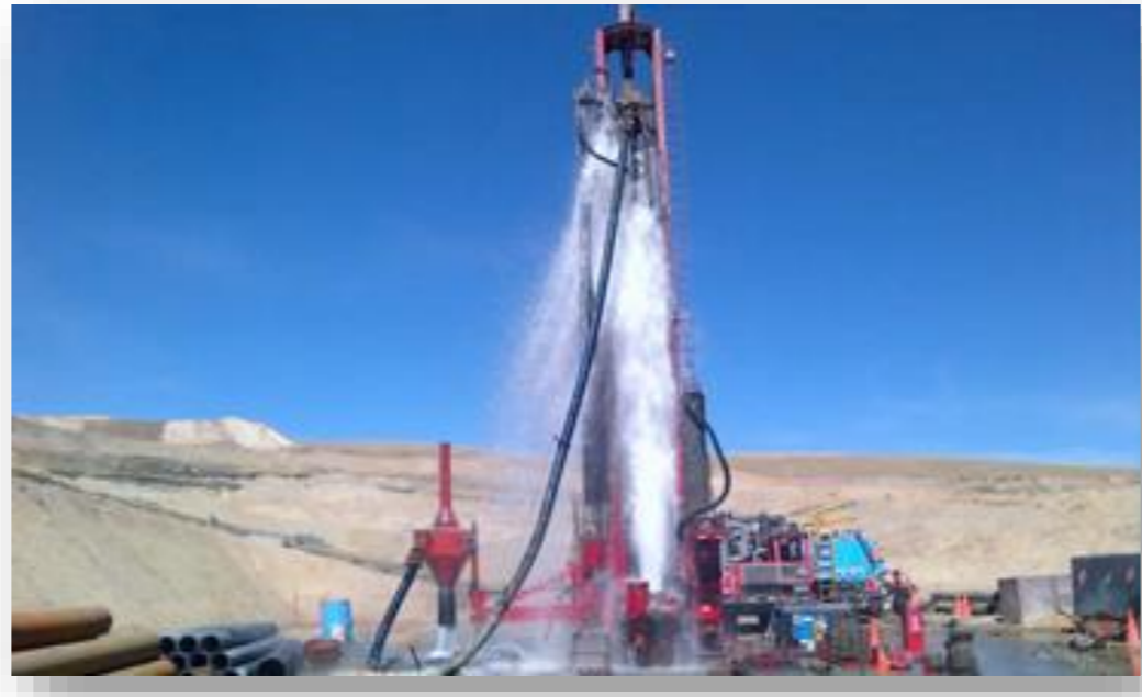
Water Well Drilling
