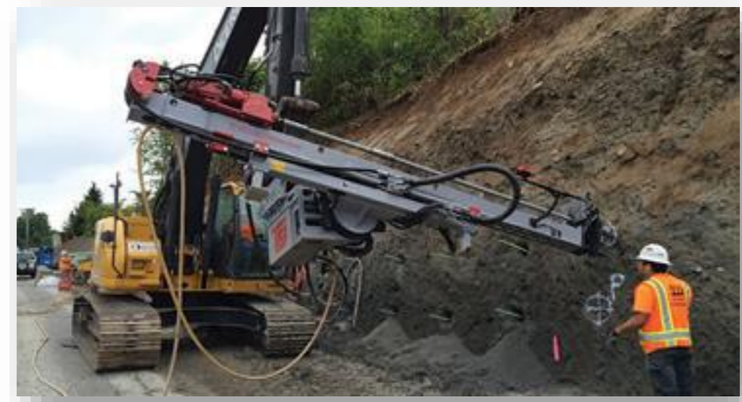
Geotechnical Drilling
